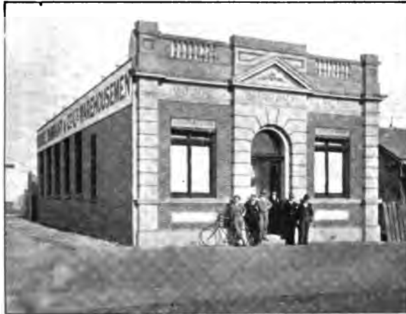
GOODE, DURRANT, & Co.'S PREMISES, KALGOORLIE.
